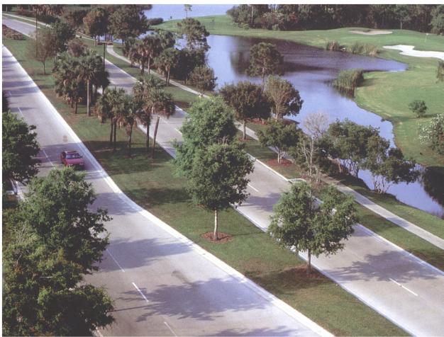
FIGURE 6.8: The steering committee selected an informal landscape theme for the parkway, with informal plant massings and naturally, random spacings.
