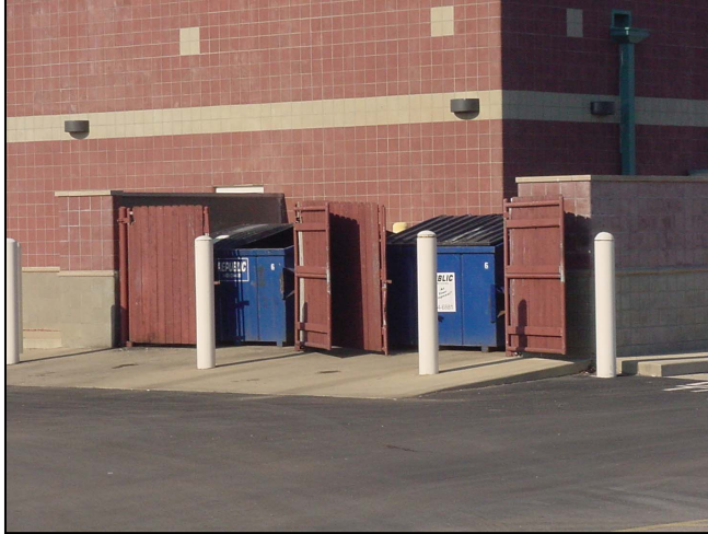
Figure 15: Screened Refuse Area
