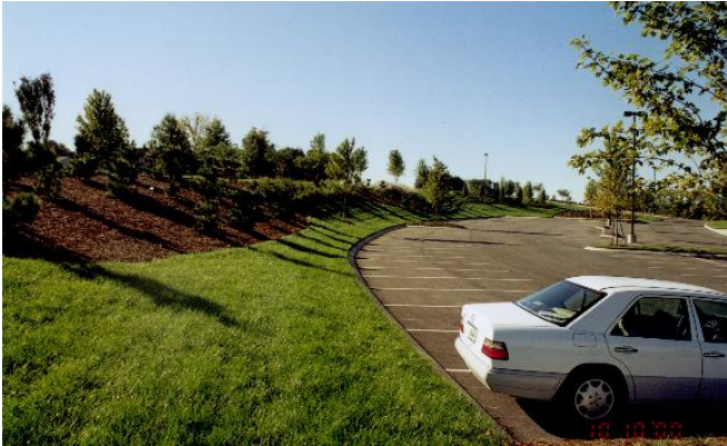
Figure 5: Example of Earthen Mound
