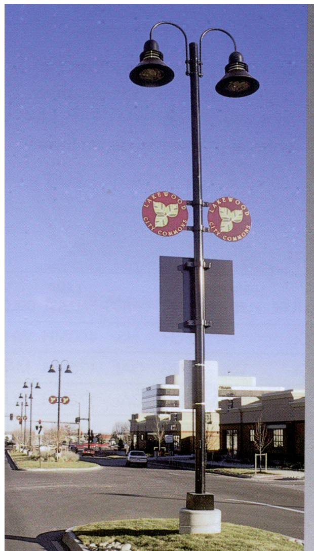
FIGURE 6.15: The preferred level of lighting enhancements for the Parkway is the use of an ornamental light with a decorative pole, decorative light fixtures, and special medallions with the parkway name or logo.
