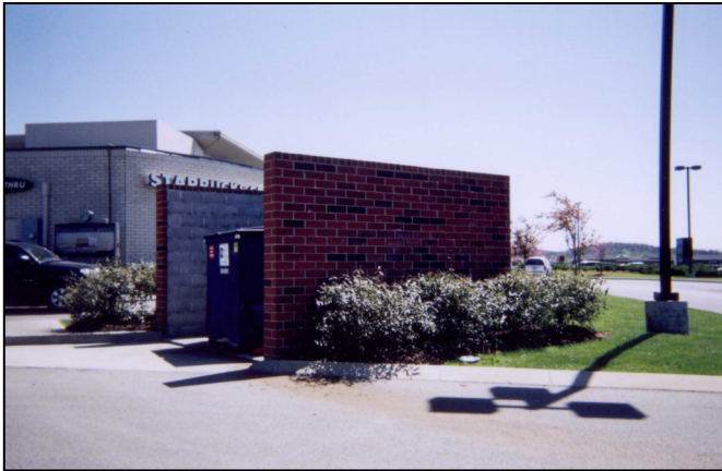
Figure 16: Screened Refuse Area
