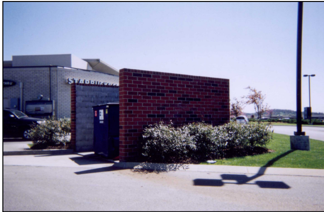
Figure 16: Screened Refuse Area
