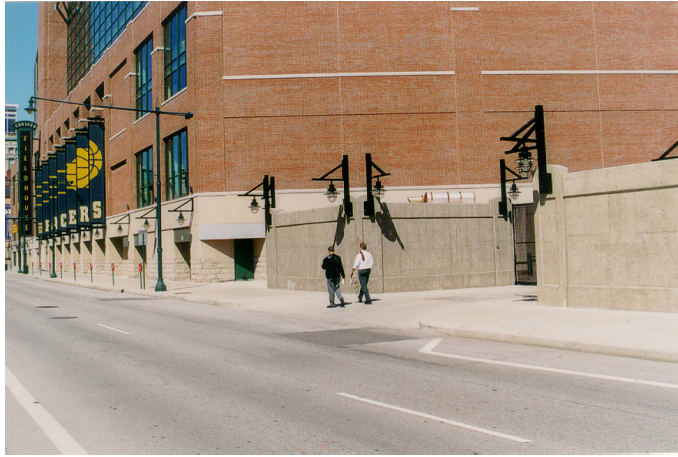
Figure 18: Example Loading Area
