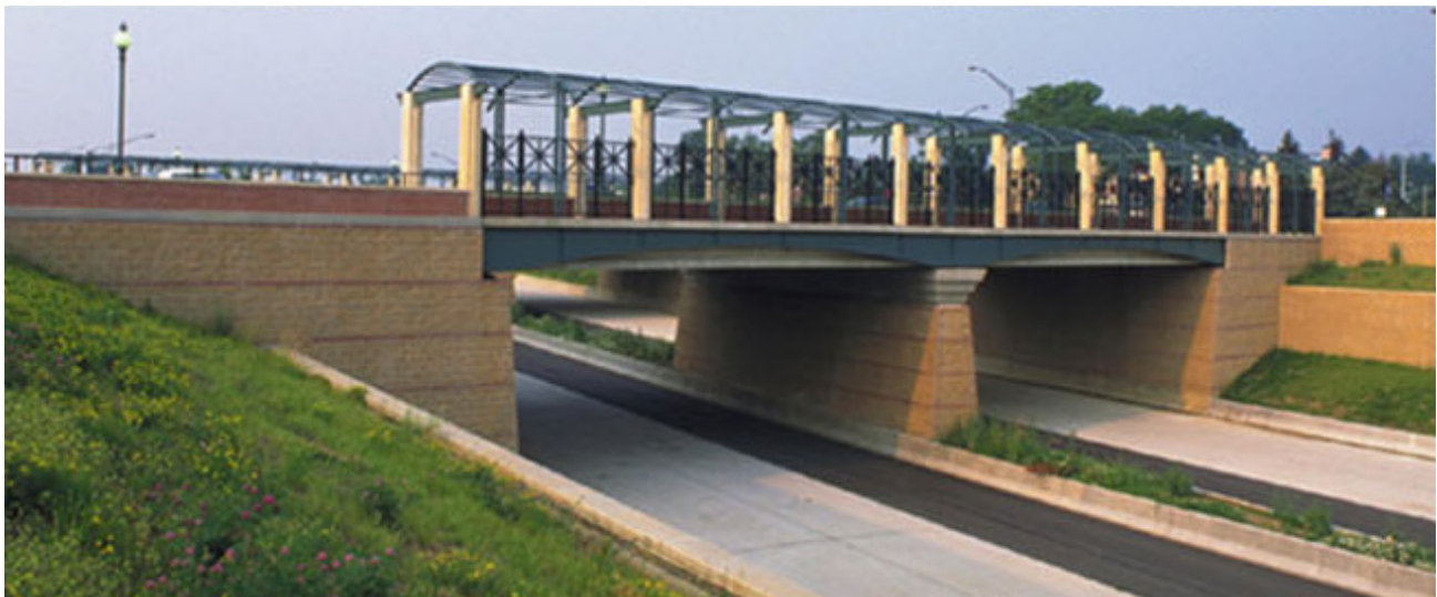
FIGURE 6.36: The image above shows enhanced treatments on bridges, a corridor aesthetic selected by the steering committee.
