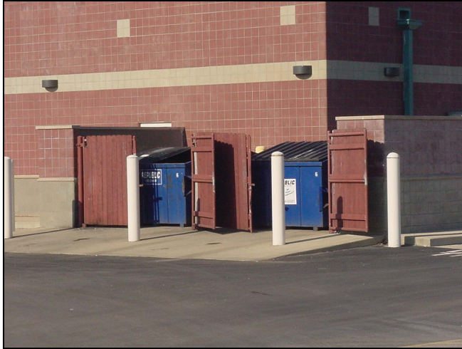
Figure 15: Screened Refuse Area
