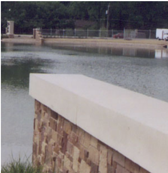
FIGURE 2.4: Limestone wall caps are used frequently throughout the City of Indianapolis as a high-quality material that is quarried locally.
