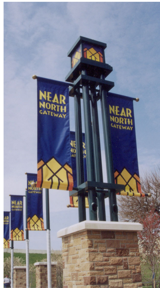
FIGURE 2.5: Limestone wall caps and sandstone veneer are utilized in Indianapolis' Near North Neighborhood to convey a classic Indiana look with modern applications.
