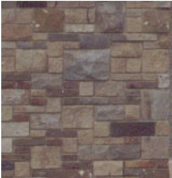
FIGURE 2.2 Ashlar sandstone veneer with machine split face in a range of colors & sizes.
